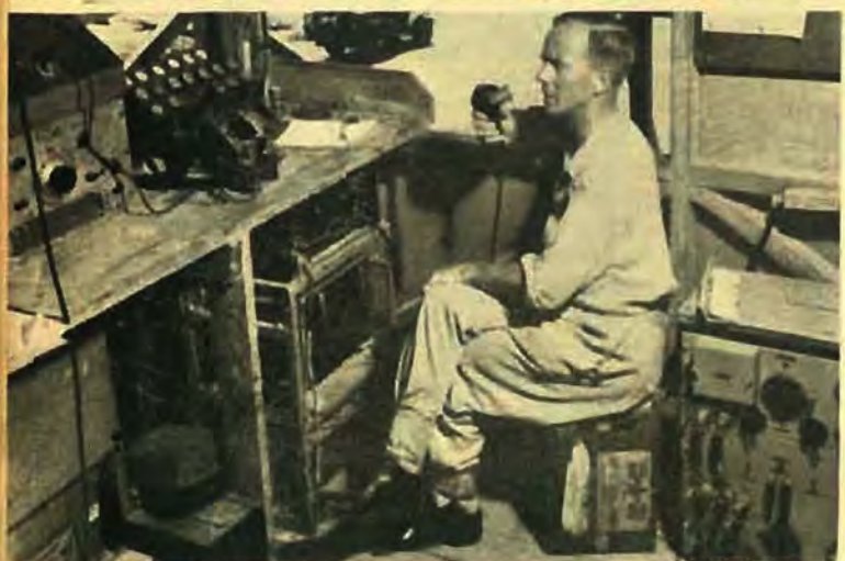
Immediately above can be seen airstrip control tower equipment used by 47 OBU at Labuan. At left is a Kingsley AR7 with VHF and HF speakers mounted above. A VHF 5043 is mounted beneath the desk, while at right is an Airzone-made BTR1, transmitter, receiver and identification equipment. The photo at top was taken from this control tower and shows three Mosquitoes flying over the strip.
