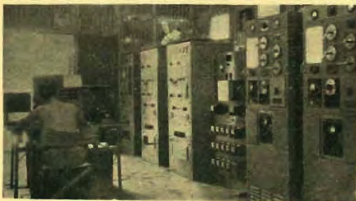
At top right is a general view of RAAF Darwin transmitting station. Top left shows the interior of the ADHQ station at Darwin with a line-up of AT5 transmitters at rear. Immediately above is the interior of the Telecom transmitting station at Darwin with two AT13's (made by AWA).
