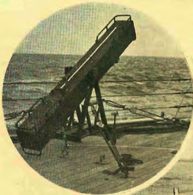
Tests of CSIR Photo-cell Chronometer on HMS King George V—quarter-deck installation on right. Inset, the rigid base sky screen.
