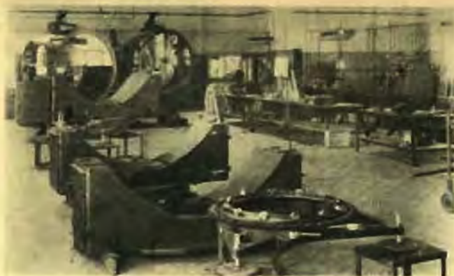
150cm. searchlight projectors in production at the Melbourne factory of A. G. Healing Ltd.
