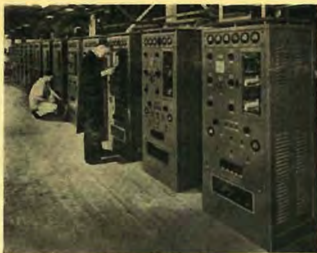
Final assembly of RAAF AT8 transmitters at STC's Sydney factory.
