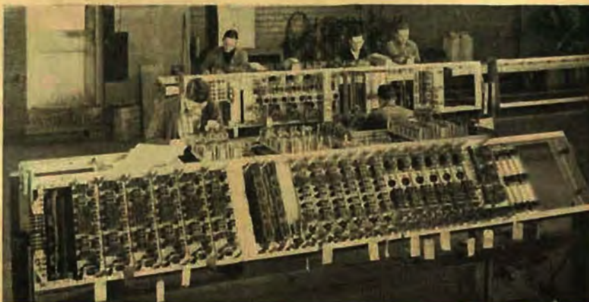
S.T.C. manufactured much carrier telephone equipment which played a highly important part in the nation's telecommunications throughout the war. Picture shows the assembling and wiring of S.T.C. Carrier Telephone and Voice Frequency Equipment.
