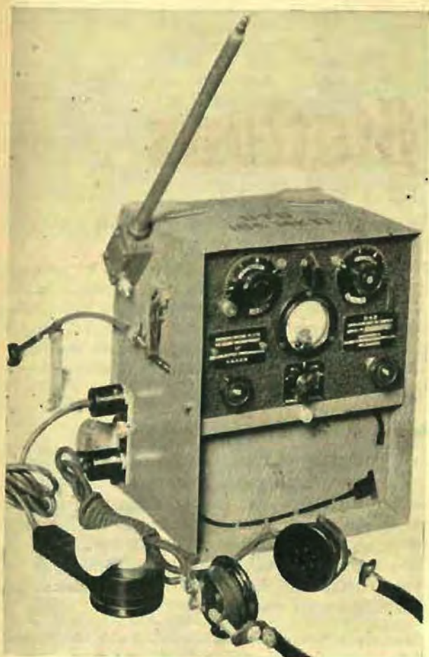
Developed for jungle warfare as a result of experience with the 108 Mk II and the 208, the Army 108 Mk III shown below was built by Radio Corporation and saw extensive service throughout the SWPA. This equipment, like the others on this page, was completely battery-operated and designed for "man-pack" operation.
