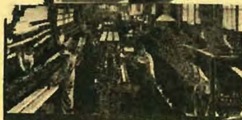
LEFT: Top and bottom boom of spar being made ready for splicing, glueing and clamping.
