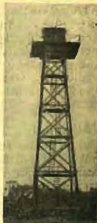
Above is a view of the plotting room at the ADHQ at Morotai. In the foreground is the plotting table and at rear two of the AR7 receivers. At right is the 70 ft. tower overlooking the perimeter, which housed the ADHQ, VHF D/F equipment.
