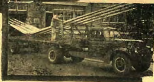
ABOVE: Finished spar loaded and ready for delivery. In a power dive at 600 m.p.h., these laminated spars were proved to retract as far as 24 inches without any structural fault developing.
