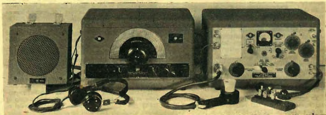
One of the later versions (the "3B2") of the AWA "Telaradio" equipment is shown below. Developed from a pre-war commercial design, this equipment saw very wide application by all Services and was used in air-warning networks, small craft and for many other purposes. The equipment normally was battery-operated and comprised separate transmitter and receiver units, covering 2.5-10 MC/s.
