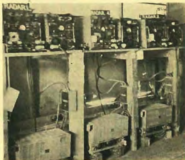
The photograph above and those below show various equipments at the RAAF Telecom Unit transmitting station at Madang. Above are three AT5 transmitters, made by AWA, with line relays for each mounted on the floor beneath each transmitter. Below, from left to right, are: 1. Two AT14S HF transmitters (made by AWA). At the left of the picture one of the station personnel is removing an STC transmitting valve from its packing case. 2. The 50 line patch panel through which all lines feeding into the transmitters are controlled; and 3. An AT17 VHF transmitter, made by Thom & Smith (left) and an AT20 (STC).
