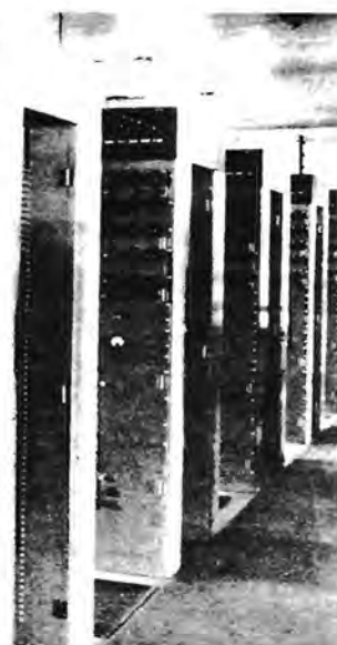
View of one section of receiver room in main shortwave receiving building of R.C.A. Communications receiving station, Riverhead, New York, showing in foreground three complete three-set diversity receiver groups and ends of 11 rows of such receiver groups.
