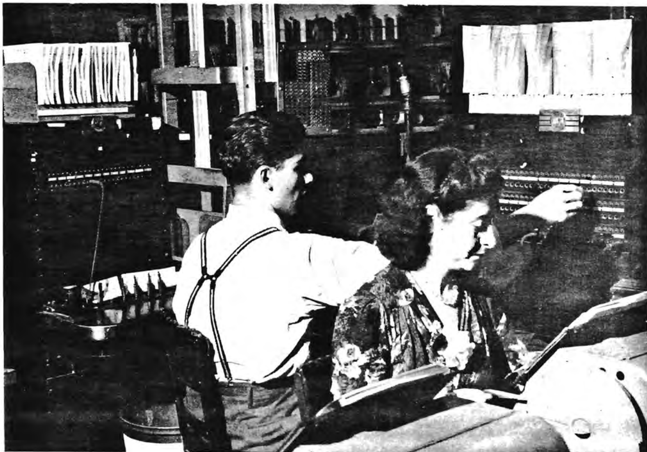
Printer concentrator switchboards controlling banks of private line customers printers. At terminal operating offices of R.C.A. Communications, New York City.
