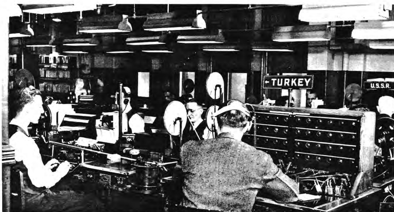
Section of terminal operating office of R.C.A. Communications, New York City. Foreground shows radiotelegraph concentrator position for switching of non-continuous circuits to active operating positions.
