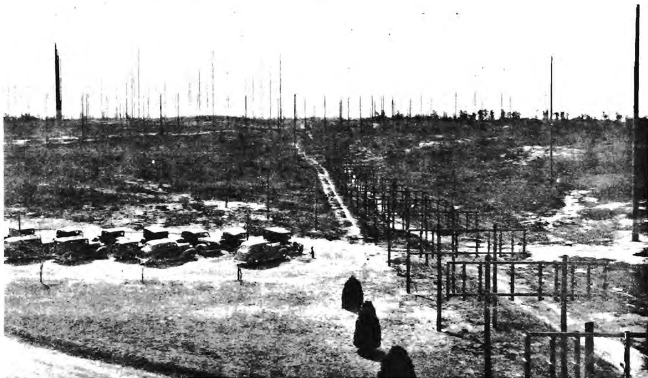
View from front of main receiving building at Riverhead showing one of the transmission line trunk systems and more of the antenna poles.
